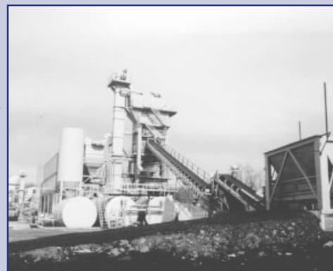
Asphalt plant in Carroll County, Maryland. Processed shingles weighed and mixed in pug mill for use as asphalt paving.
