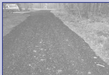
Course-ground shingles used as a driveway.
